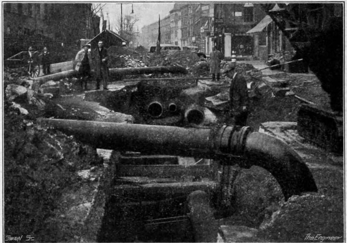
12-INCH RIDER WATER MAIN JOINING ENDS OF 24-INCH MAIN
