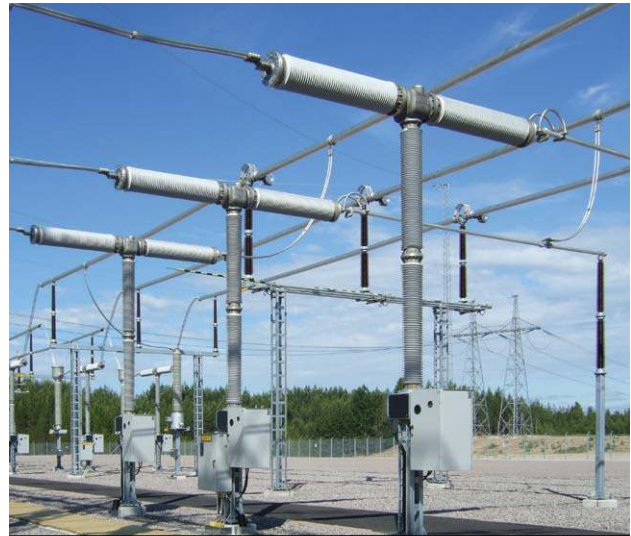
Disconnecting circuit-breaker. Same contacts for switching and disconnecting functions.
