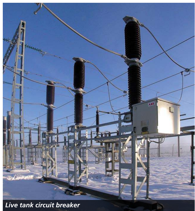
Disconnecting circuit-breaker. Same contacts for switching and disconnecting functions.
