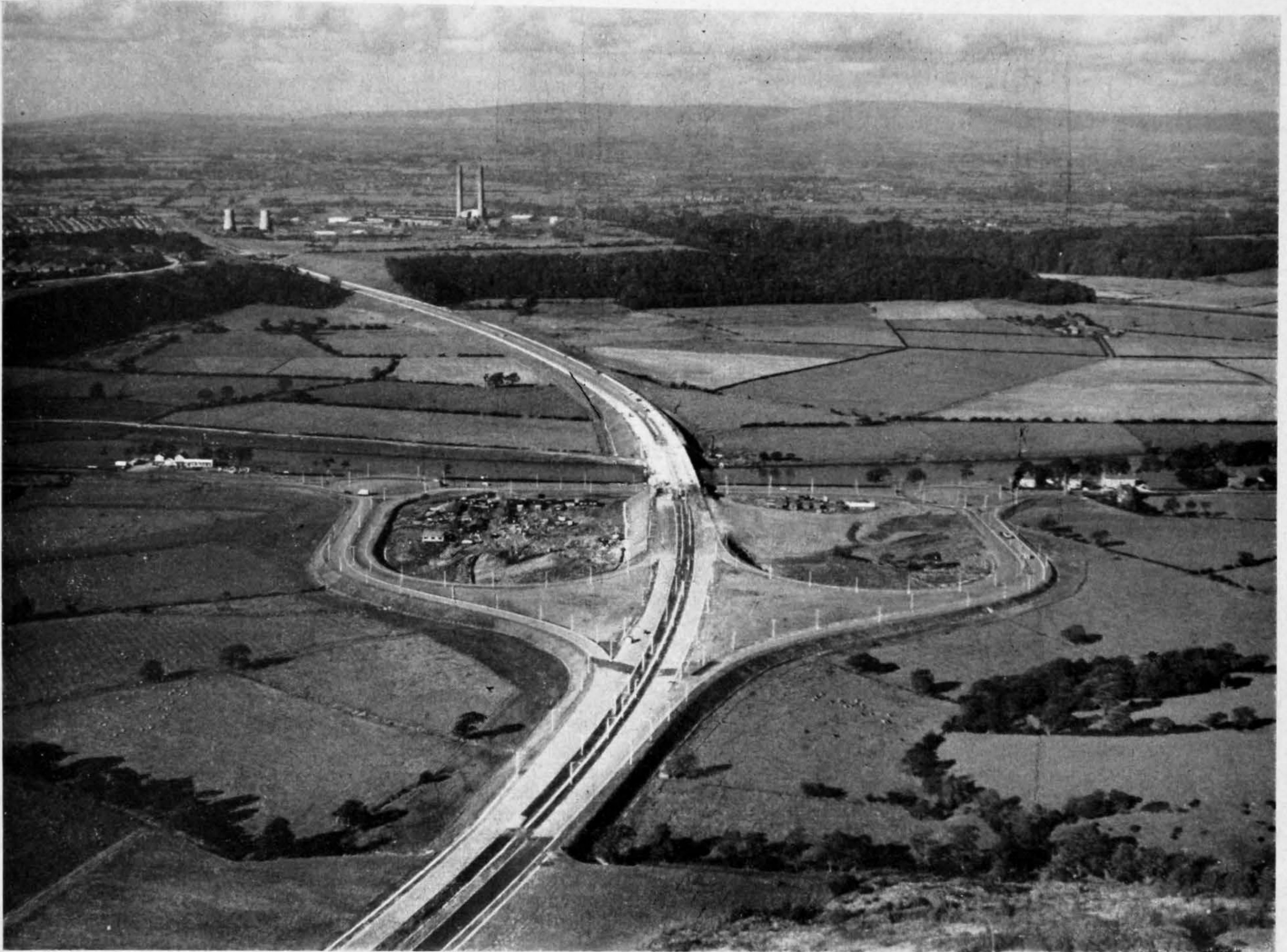
The Preston by-pass motorway at the junction with the Preston-Whalley road. At this point the motorway crosses the River Ribble and sweeps away to the northward
