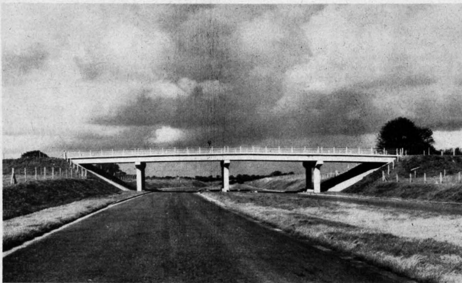
Broughton Hall bridge carries a Class III road over the motorway, the spans being 36ft 6in, 49ft, 49ft and 36ft 6in. The width of the bridge is 34ft, piers and abutments are on concrete piles and the deck is of precast prestressed concrete beams
