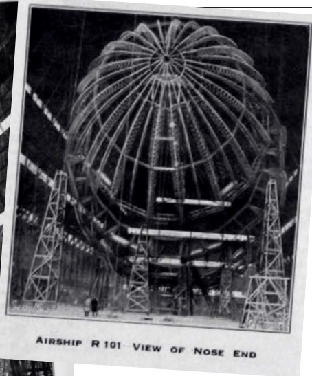
↑ The R101 airship, in which Lyon played a key role, taking shape at the Cardington airship works. Image: The Engineer
