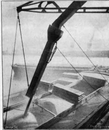
FIG. 2—DISCHARGING GRAIN INTO BARGE
