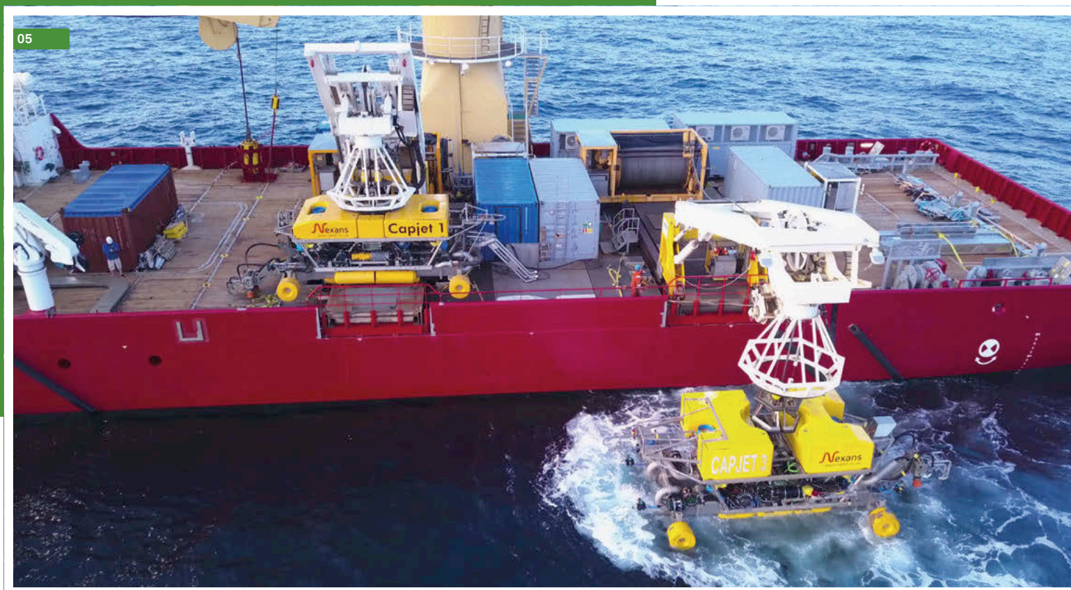
05 A range of specialist vessels and ROVs are used to install subsea cables
