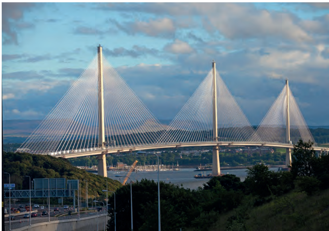
The £1.35bn Queensferry Crossing spanning Scotland's Firth of Forth has opened to traffic for the first time. At 2.7km in length, the new structure is the longest three-tower cable-stayed bridge in the world.
