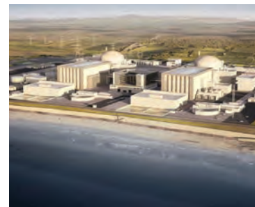
Hinkley Point C in Somerset
