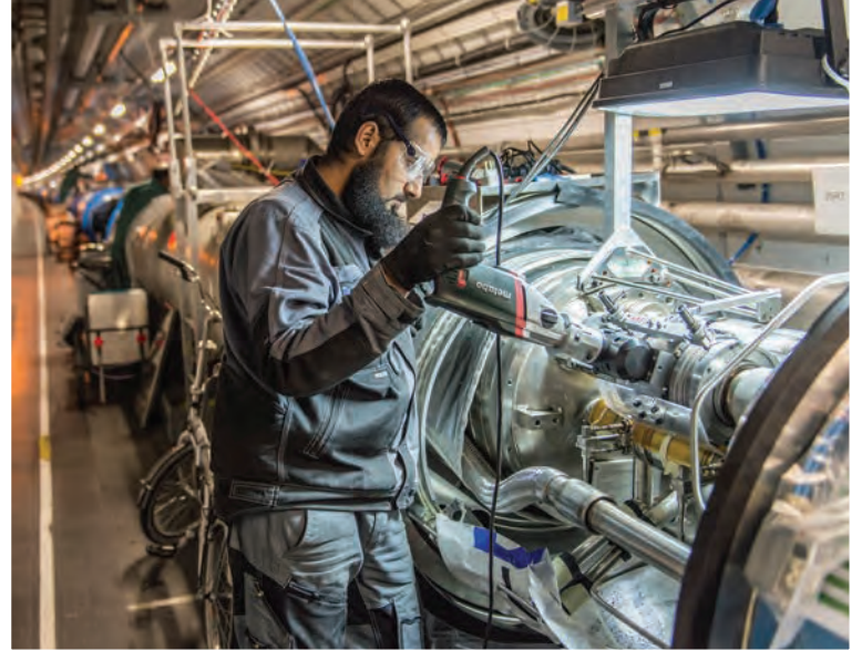
Above: the upgrade of the LHC doubled the energy available for experiments Below: welding around the LHC's superconducting magnet channels
