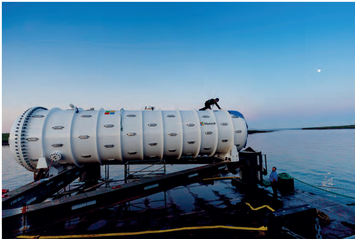
Spencer Fowers, senior member of technical staff for Microsoft's special projects research group, prepares Project Natick's Northern Isles data centre for deployment off the coast of the Orkney Islands in Scotland. The data centre is secured to a ballast-filled triangular base that rests on the sea floor, with seawater helping to cool its servers.
