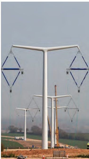
The newly introduced 35m-tall T-pylons
