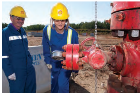
Left to right: an absorber tower; the Goldeneye platform; a CO 2 stripper at Canada's boundary dam CCS project; and a CO 2 injection well on the Quest project
