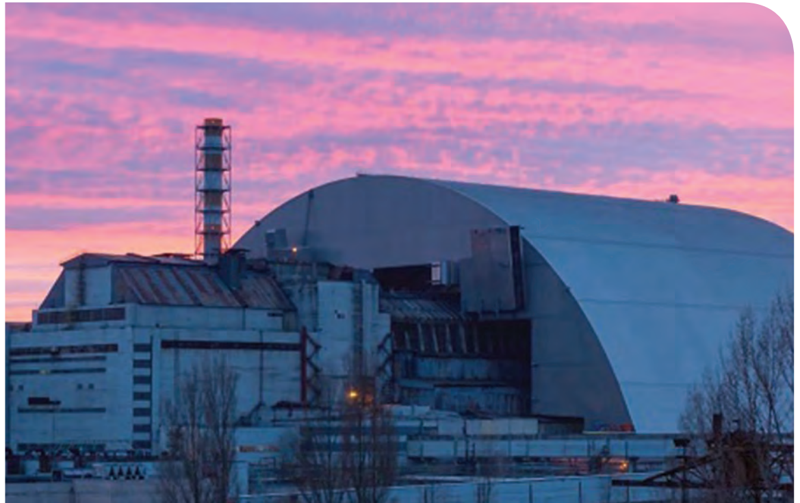
The radioactive remains of Chernobyl's Reactor 4 have been safely enclosed after moving the plant's New Safe Confinement (NSC) over a distance of 327m from its assembly point to its final resting place. The NSC completely encloses a previous makeshift shelter that was assembled immediately after the 1986 accident.
