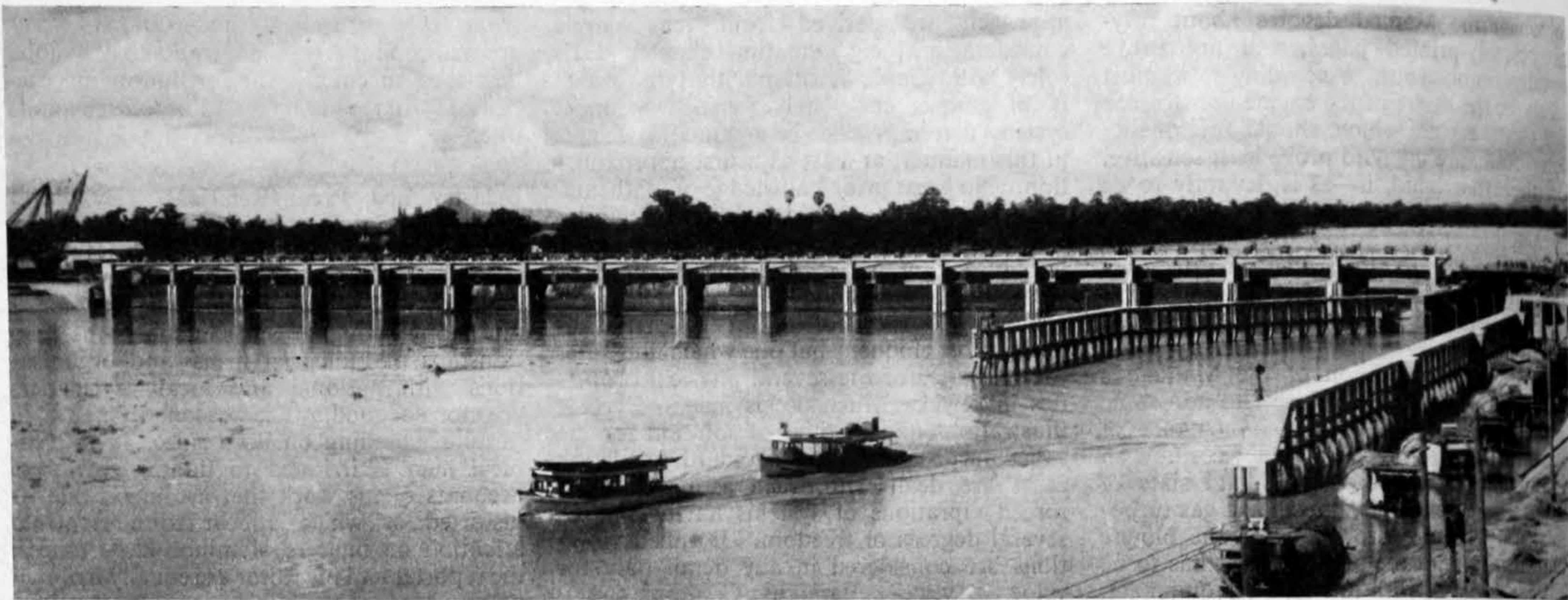
The completed Chainat barrage from upstream. The approach jetty for the lock is shown in the foreground with the sector gates and the bridge for the gates operating machinery further back
