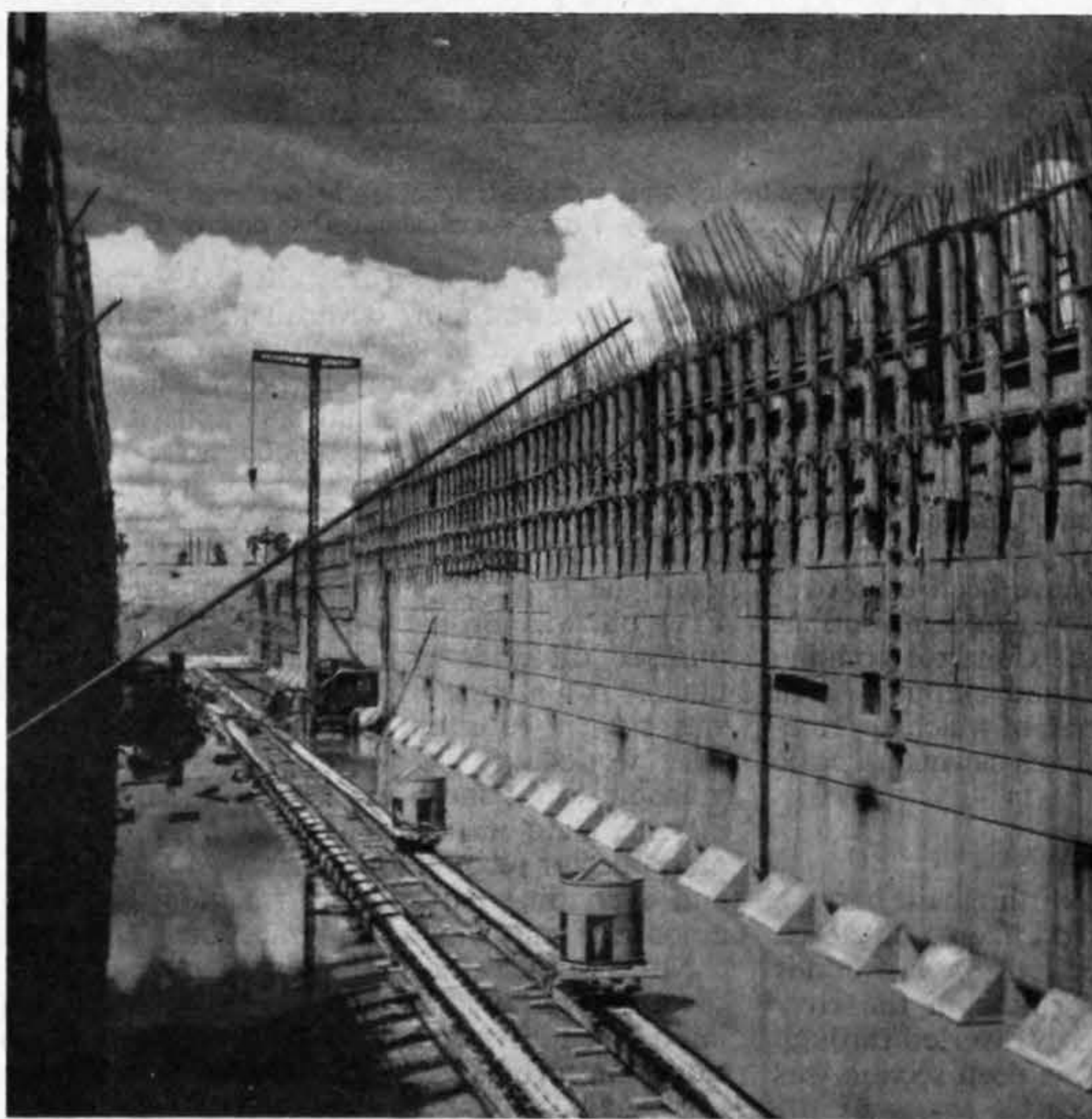
Construction of the lock in progress. Note the 6-ton crane with a 50ft jib made on the site
