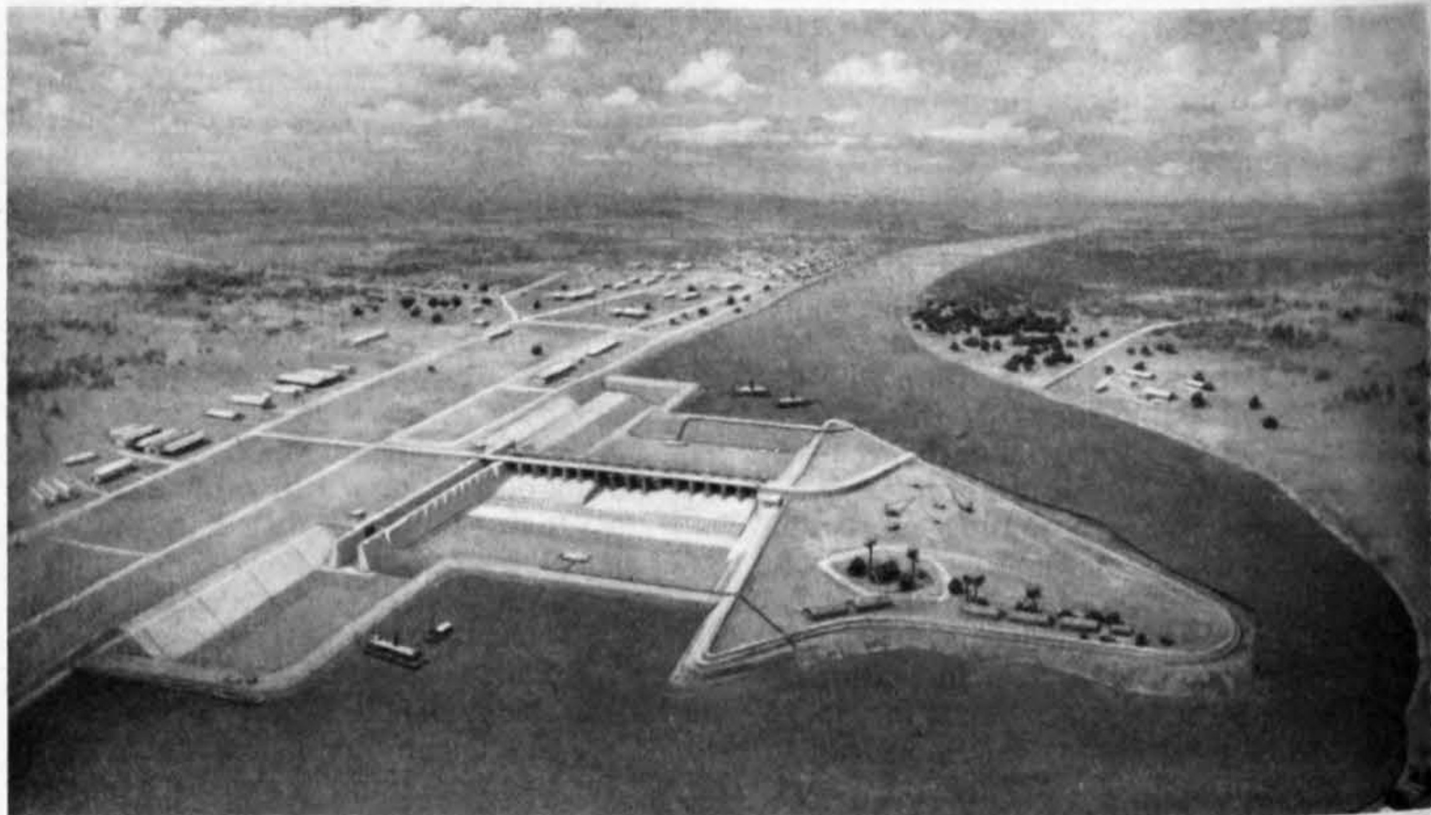
Diorama of the Chainat barrage. The stage shown is with the main works complete, but with the dam still "in the dry" as during construction. To complete the work, the cofferdams were dug away, and an earth dam built across the river, between the bunds shown on the right. Note the discharge points from the well-point drainage.
