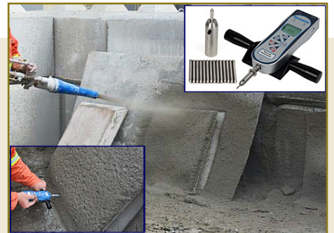
Spraying a sample and early strength testing with a digital penetrometer
